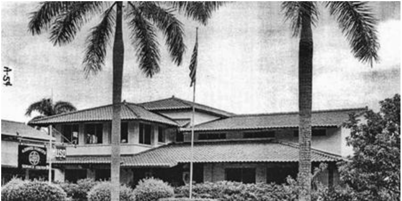
The USO-Jewish Welfare Board building, aka Jewish Welfare Center, at La Boca Road before the crash. Across the street was St. Mary Catholic Church. On the east side of the building was the Elks Club and then the Balboa Police Station on the corner of Amador Road. Photo submitted by Michael Witkin.
