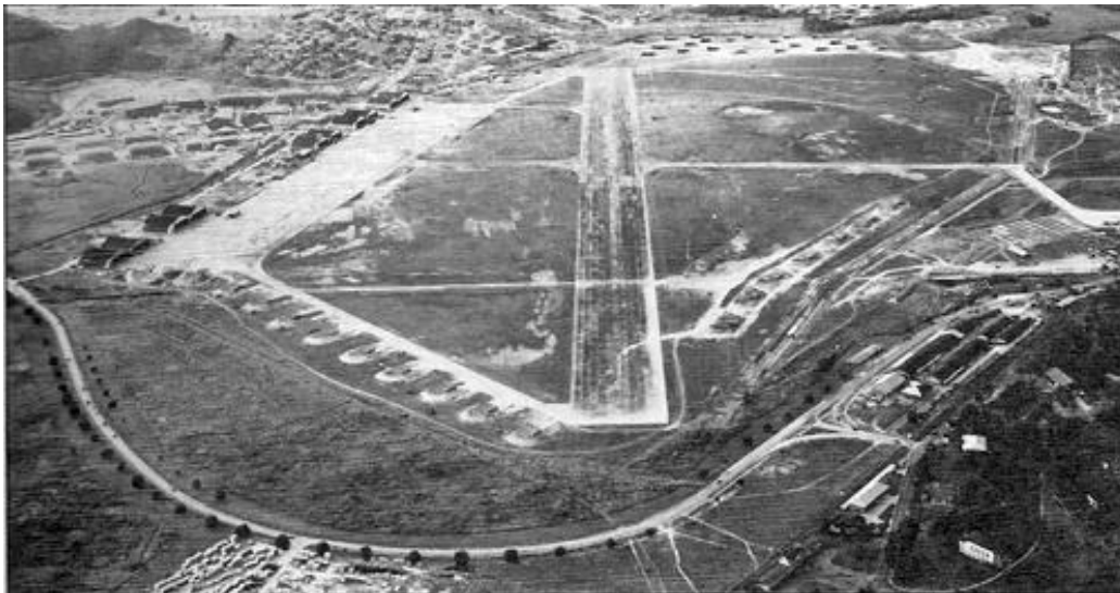
Albrook Field looking north, February 11, 1942. Note revetments built to protect the individual planes from enemy attack. Photo from "Wings Over The Canal".
